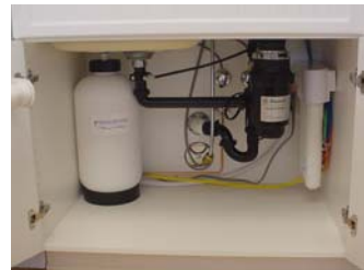
EWA BEACH (Ocean Point) Installed 3/3/05
