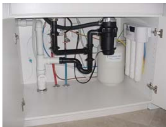
Ewa Beach (Ocean Point) Installed 6/21/07
