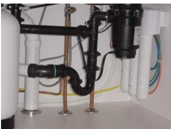
EWA BEACH (Ocean Point) Installed 2/2/05
