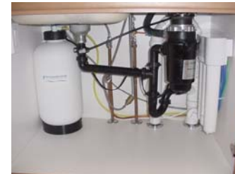
EWA BEACH (Ocean Point) Installed 11/10/05
