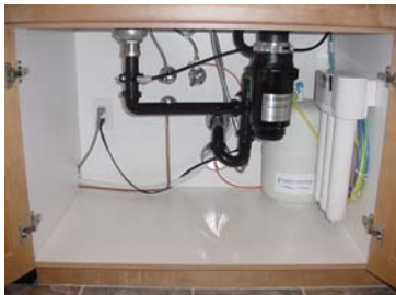
Ewa Beach (Ocean Point) Installed 9/12/07
