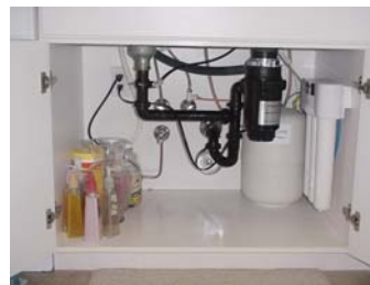
Ewa Beach (Ocean Point) Installed 6/29/07
