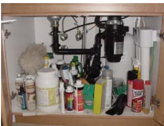
EWA BEACH (Ocean Point) Installed 9/20/04
