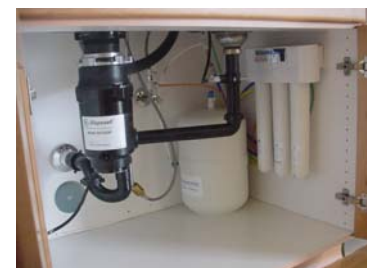
EWA BEACH (Ocean Point) Installed 6/25/08
