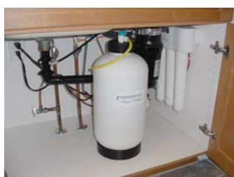
EWA BEACH (Ocean Point) Installed 8/19/05
