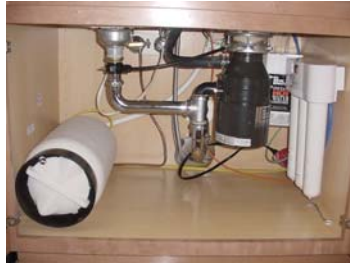
KAPOLEI (Kekuilani Palms) Installed 10/5/05
