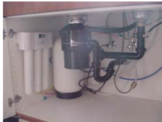
EWA BEACH (Ocean Point) Installed 10/16/04
