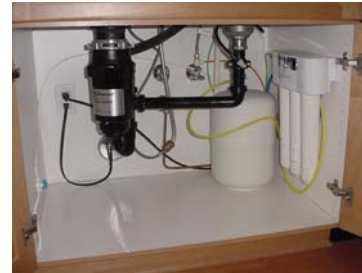
Ewa Beach (Ocean Point) Installed 8/17/07
