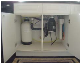
EWA BEACH (Ocean Point) Installed 7/1/04
