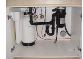
EWA BEACH (Ocean Point) Installed 7/1/04
