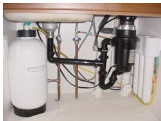
EWA BEACH (Ocean Point) Installed 5/17/05
