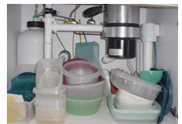
KAPOLEI (Kekuilani Palms) Installed 3/19/04
