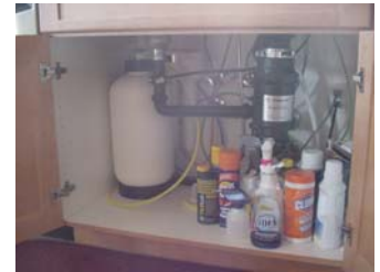
EWA BEACH (Ocean Point) Installed 2/23/04
