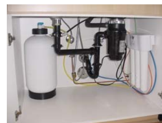
EWA BEACH (Ocean Point) Installed 9/19/05
